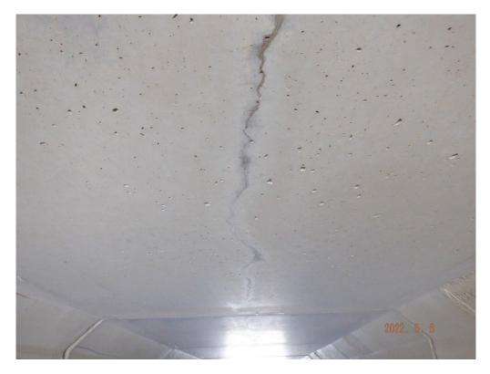
Narrow moisture crack in soffit
